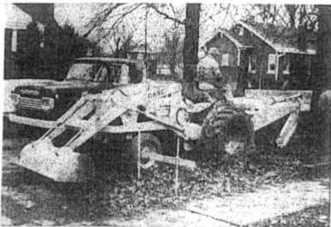
Implementing its new policy of putting in storm sewers wherever the residents are willing to pay for the pipe, the City of St. Matthews last week was busy digging in 250 feet of 18-inch and 12-inch pipe on the east side of Baser Avenue south of Wilmington. The pipe cost the residents $648. The dump truck, and the new Case grader and trench-digger (operated by Norvin Orr) belong to the City. Mayor Bernard Bowling is at right.
